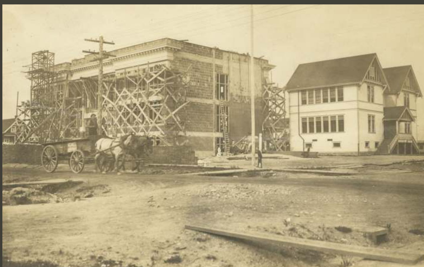
Gilmore Avenue School under construction, 1915.
